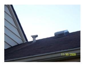
These pipes may be the flue vent for the fireplace. If so, this pipe is NOT suitable for fires. DO NOT use.
