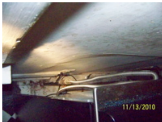
No gas valve or anti-tip bracket at stove
