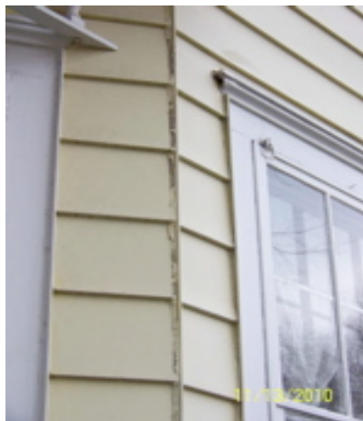
poor caulk at joints
