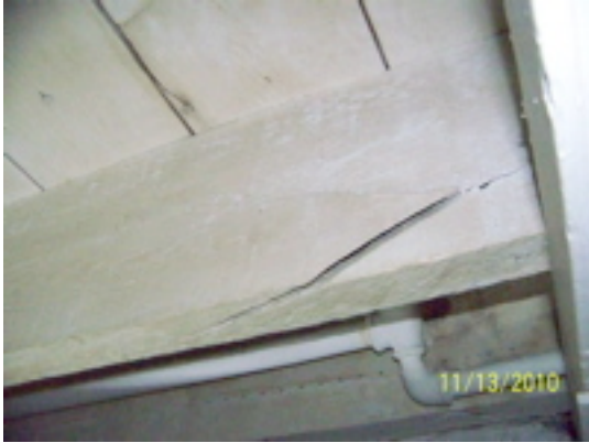
Broken joist, left of wash machine
