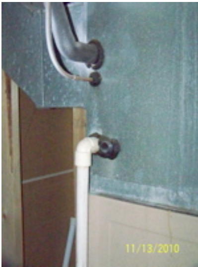
AC drain connection
