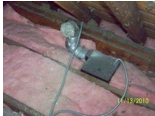
2 nd floor bath exhaust fan vented into attic
