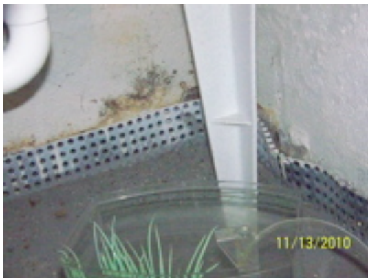
Northeast corner water intrusion
