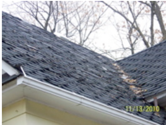
Deteriorated, curling roof shingles, front and rear roof areas
