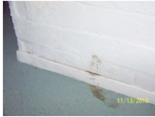
Signs of water intrusion, basement wall
