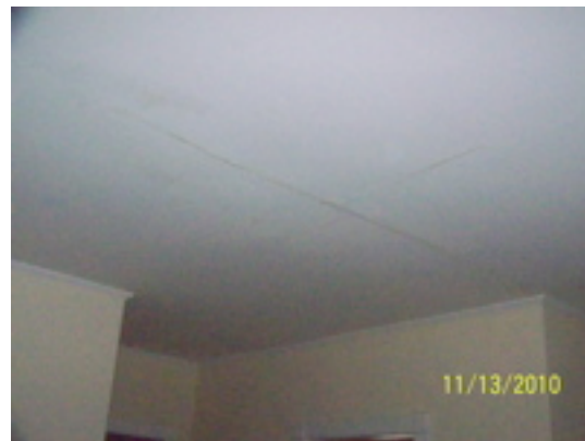
1 st floor ceiling, water damage
