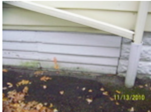
High driveway and rotted wood siding
