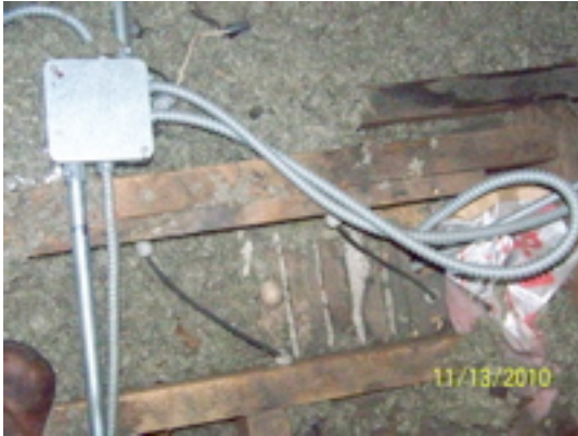
Exposed attic wiring, poor insulation
