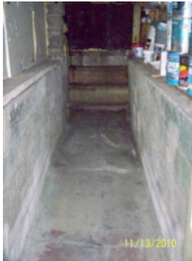
Rear retaining wall severely crack, eroded Separated and leaning in 1.25" +
