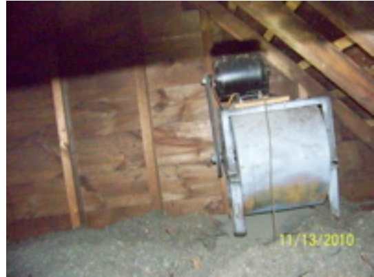
old exhaust fan in attic
