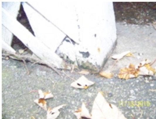
Rotted wood post base in contact with ground
