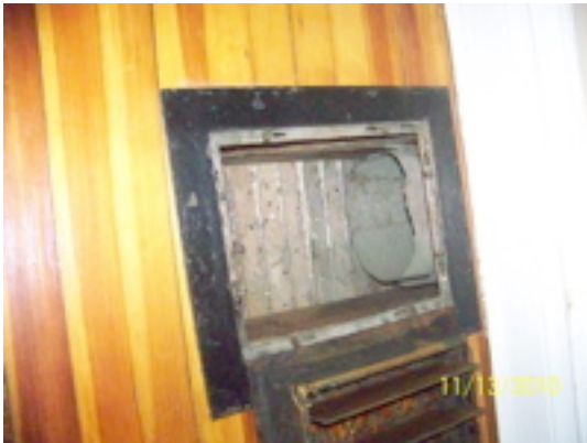
open ended duct run inside of joist cavity, substantial heat loss
