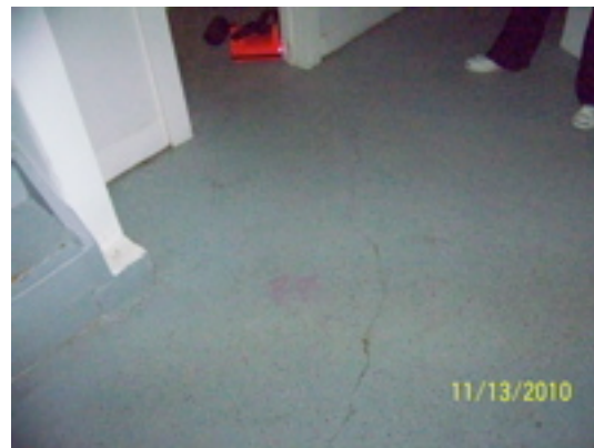
cracked, heaved floor at bottom of basement stairs. Likely due to sewer tile failure
