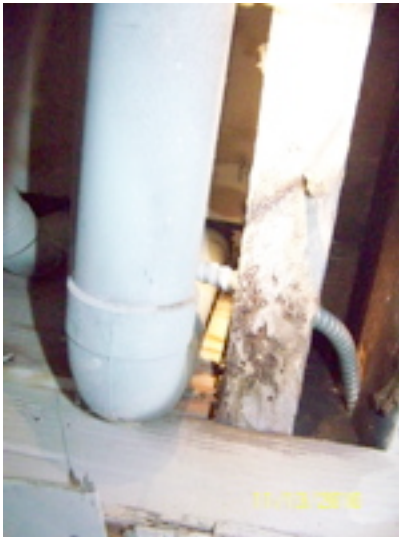
Rotted, twisted joist
