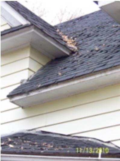
Deteriorated, curling roof shingles, front and rear roof areas
