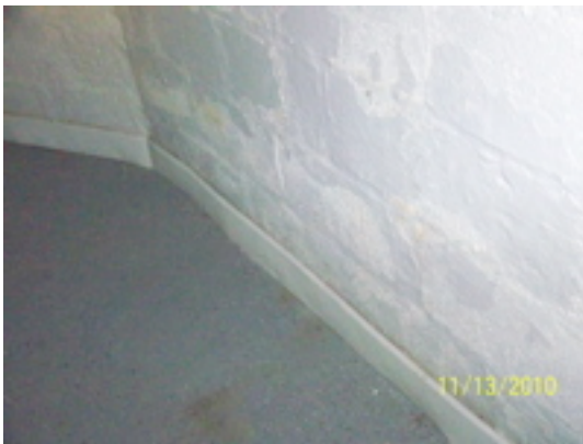
flaking paint and mortar along basement wall, typical of water intrusion
