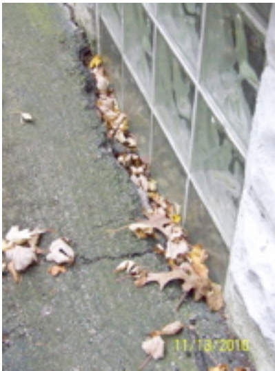
Driveway above bottom of window and top of foundation
