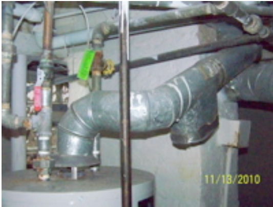
improper and hazardous flue pipe set-up for water tank
