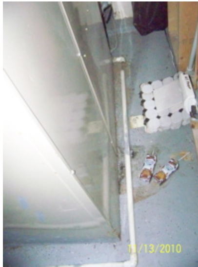
AC broken drainpipe
