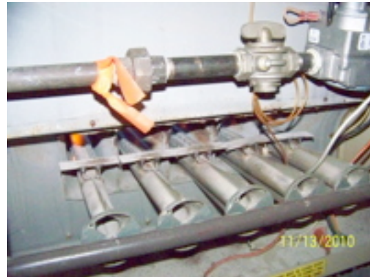
rusted furnace, jumped wiring
