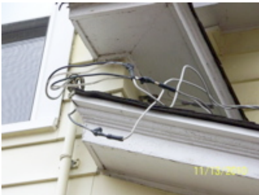
electrical service in contact with roof
