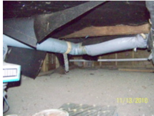
Un-insulated and not properly supported duct runs in crawlspace
