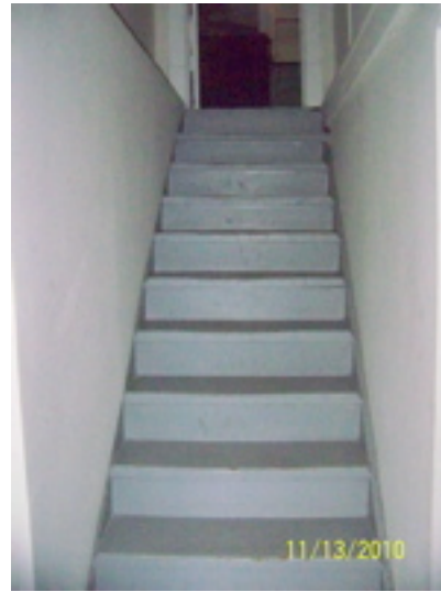
No handrail at stairs to basement
