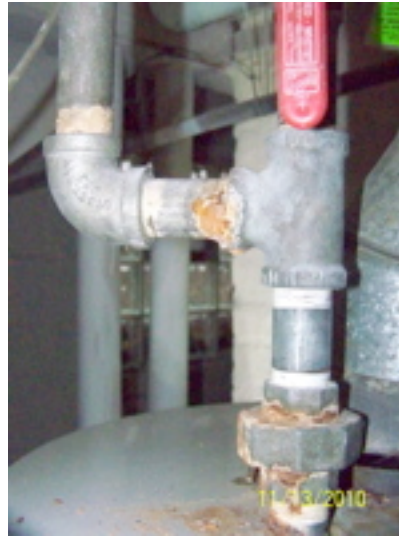
rusted galvanized pipe and fittings
