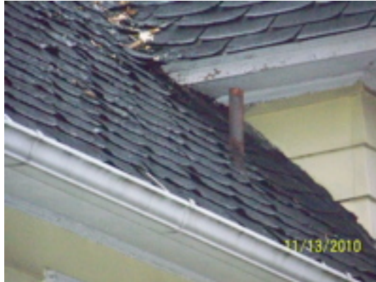
Exterior fireplace flue pipe
