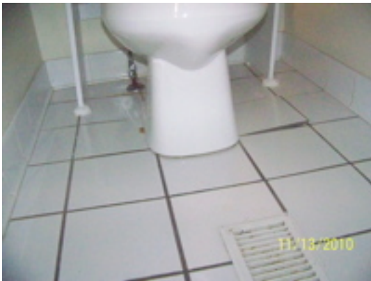
2 nd floor toilet sinking into floor tiles popping up
