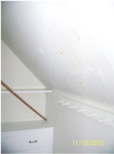
Damaged plaster from water leaks 2 nd floor front closet
