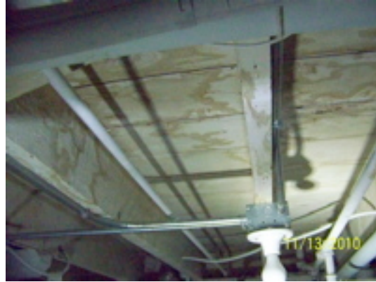
extensive water stains/damage At basement sub-floor and joists
