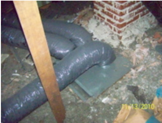
Attic duct runs, main chase and cover not insulated
