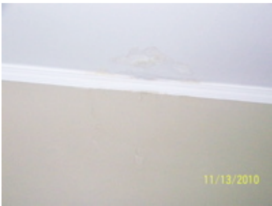
wall and ceiling roof leak damage
