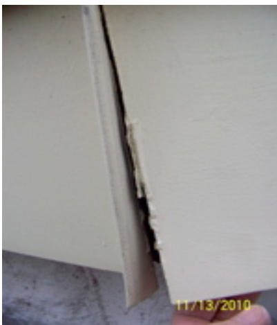
deteriorated siding condition
