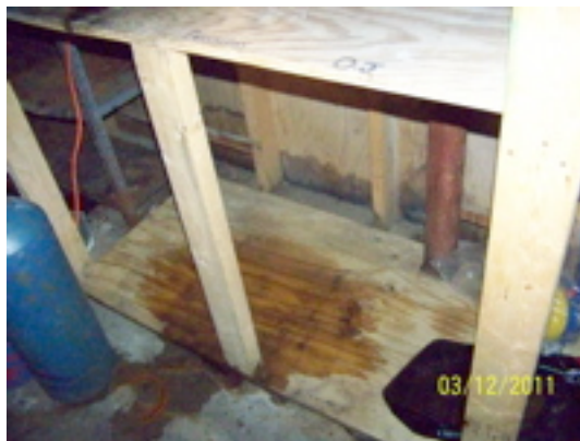
Typical water damage in basement and active water leak
