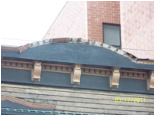
Top of east wall, missing, rotted trims
