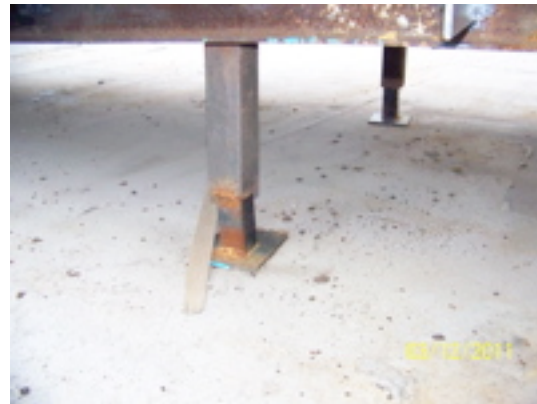
Walkway feet sitting directly on Roofing material
