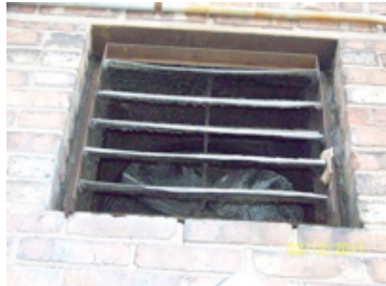
Typical through wall fan Vanes do not close fully
