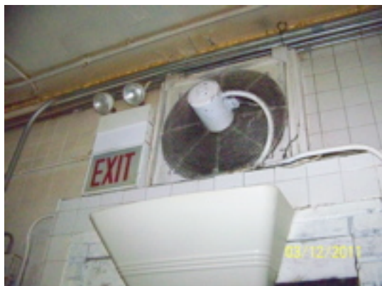
Kitchen exhaust fan, dirty Leaking air
