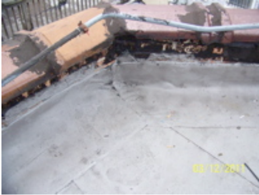
No term bar for roofing at parapet
