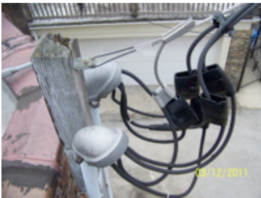
Service within reach of stair landing
