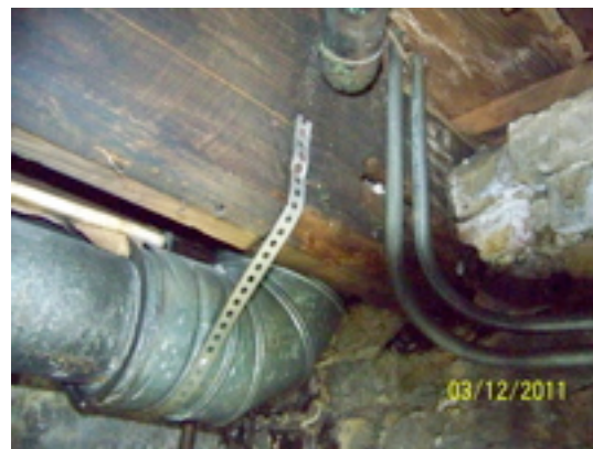
Typical rotted and cracked joists
