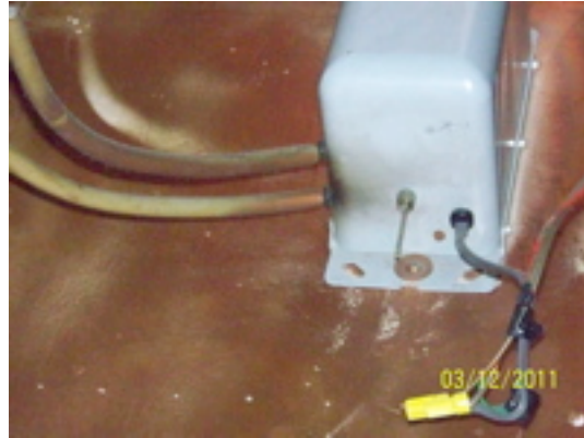
Scorched wires at transformer
