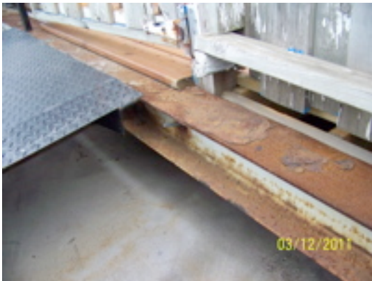
Rusting I-beam for deck support
