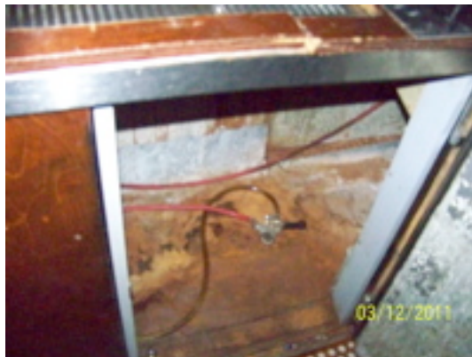
Typical rusted out bar coolers, 1 st and 2 nd floors
