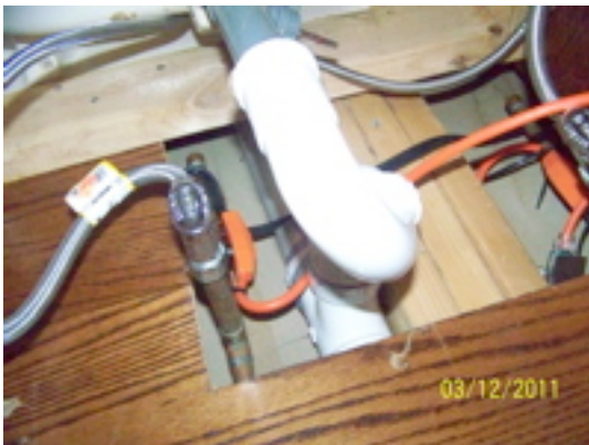
Extension cord, heat tape at pipes Under 1 st floor men's sink
