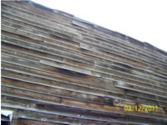
Top of south wall, rotted and open
