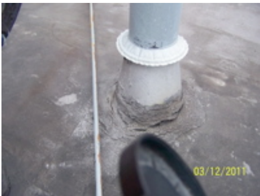
Typical deteriorated vent flashing
