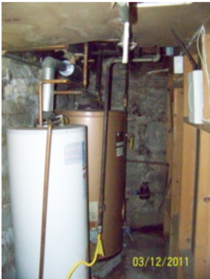
Water tanks, rear unit not Functional
