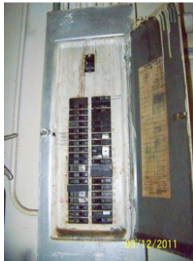
1 st floor panel, open slots
