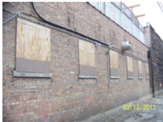
Rotting plywood at boarded windows
