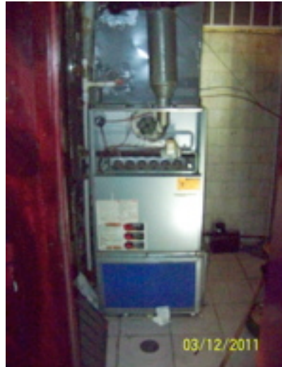
2 nd floor unit, pulling return air from closet and in front of floor drain
