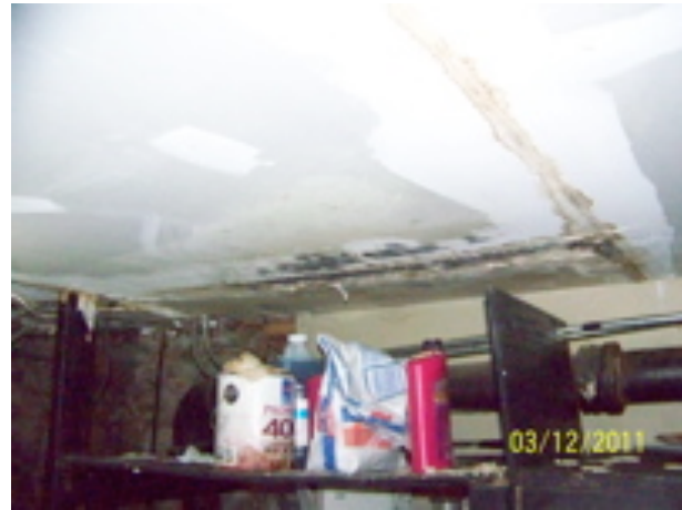
Basement ceiling water damaged drywall and joist damage
