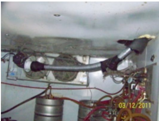
Homemade AC to 1 st floor beer tap station
