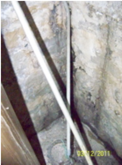
Typical wall seepage signs
