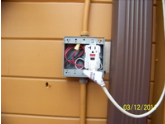
Open exterior electrical box
