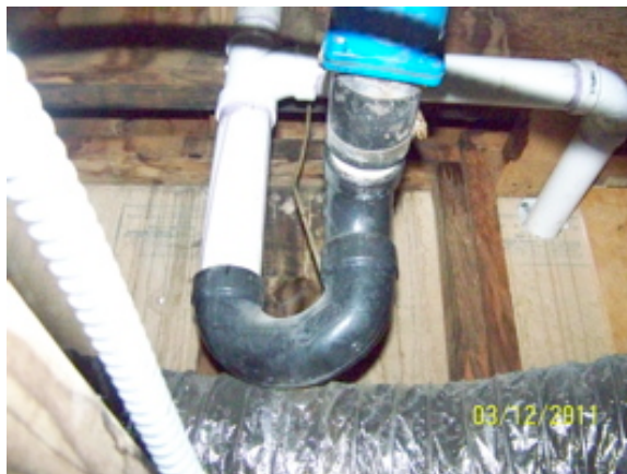
PVC and ABS drain pipe, and check valve in bathroom ceiling
