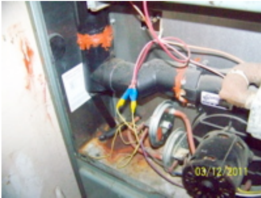
1 st floor front furnace, water damage and rust at unit cabinet
