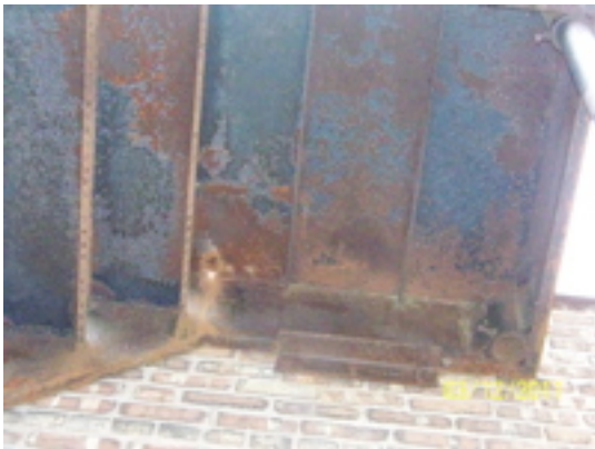
Extensive rust at rear steel staircase
