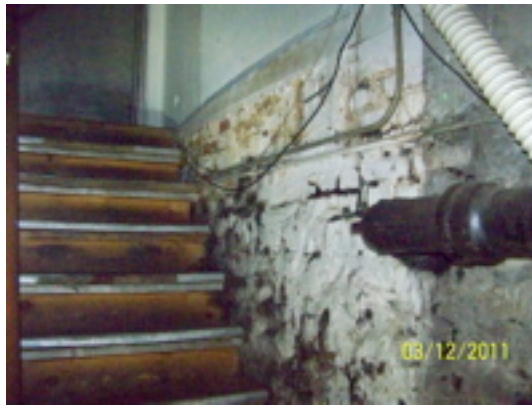
Seepage and mold signs at north wall
