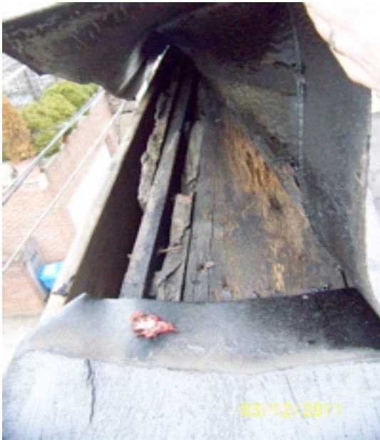
Top of 2 nd floor parapet wall rotted out
