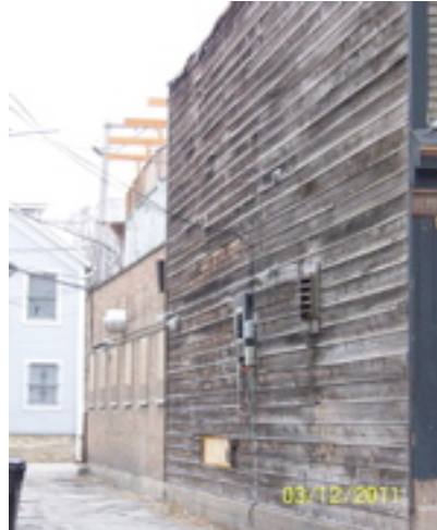
Main south wall, rotted and open
