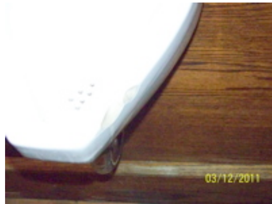
Porcelain chips on 1 st floor urinal
