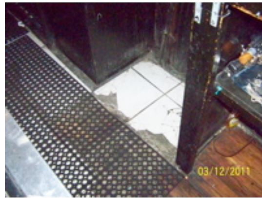
Rotted, unstable floor behind 1 st Floor bar area
