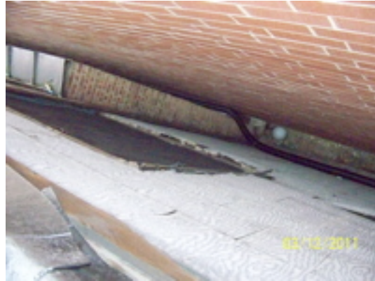
Open and broken areas on north wall
