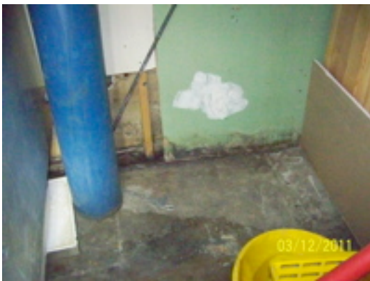
Typical water damage in basement and active water leak
