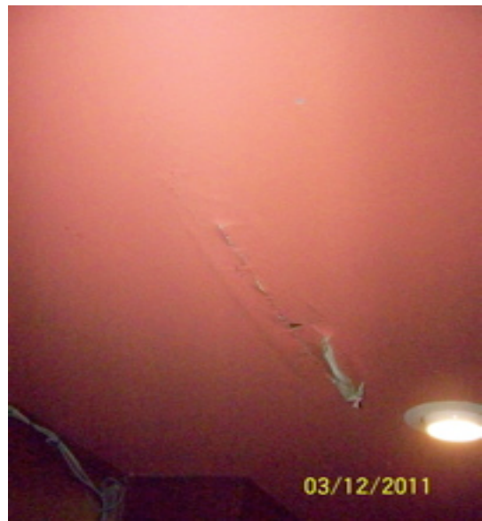
2 nd floor ceiling roof leak signs
