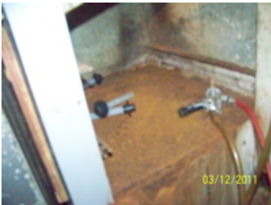
Typical rusted out bar coolers, 1 st and 2 nd floors
