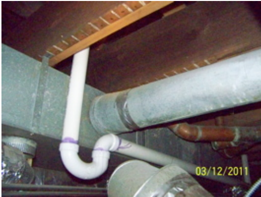
2 nd floor PVC floor drains
