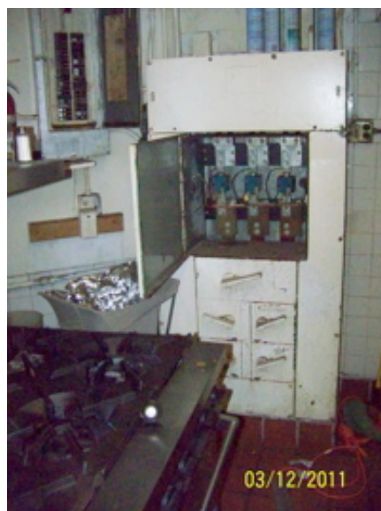
Live buss, main switchboard 1 st floor kitchen
