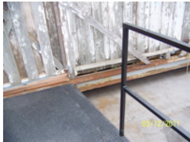
Missing guardrail, 2 nd floor egress
