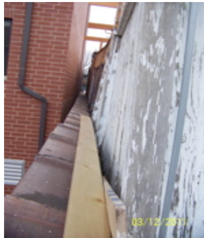
Rotted and leaning walls At 2 nd floor deck
