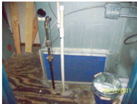
Unit pulling return air from furnace closet
