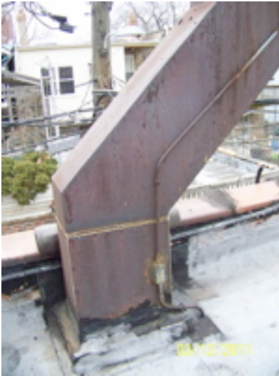
Rusting duct for main Kitchen exhaust hood
