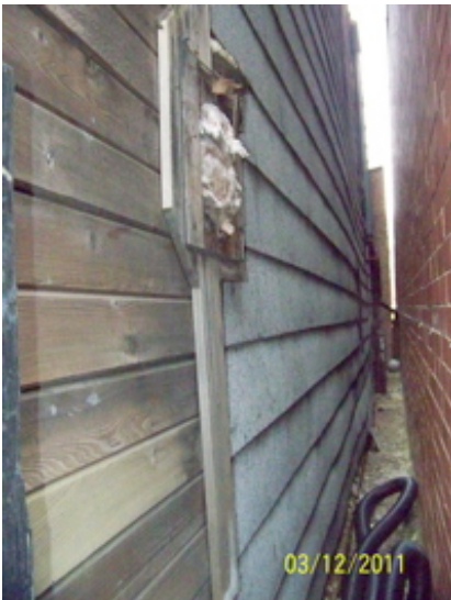
Hole in north wall, poor siding
