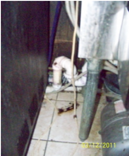
PVC drains at bar sinks
