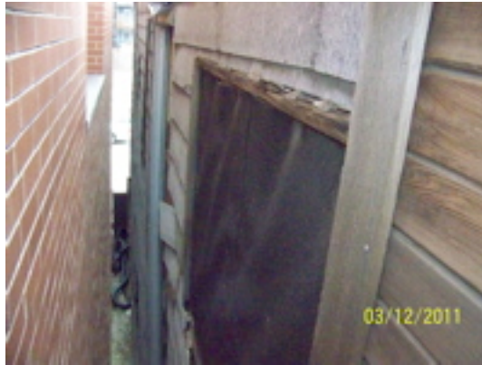
Open north wall allowing water intrusion
