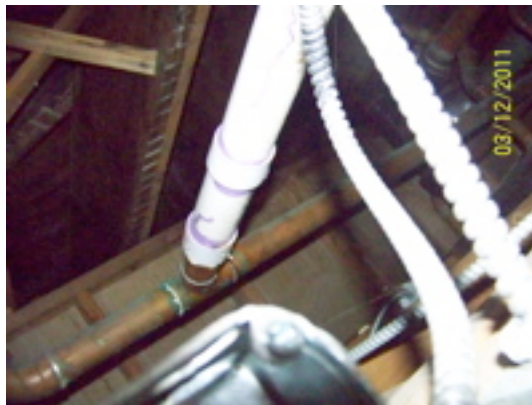
PVC drain tied into copper run
