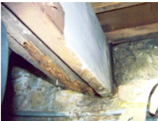
Typical rotted, un-supported joists
