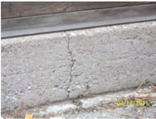
Typical foundation wall cracks
