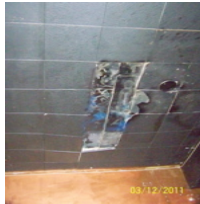
Damaged seating area and hanging ceiling tiles, 1 st floor rear bar area
